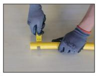
Cut the plastic cover on the inflex hose (as the 6th node is outside) with a scraper tool. 2-(by turning around the hose) Then remove the plastic cover by cutting parallel to the axis of the hose with a utility knife.
