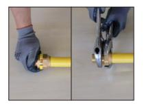
5-Screw the nut onto the body by hand first and take the gap. Then fix the body and screw the nut with a wrench.
